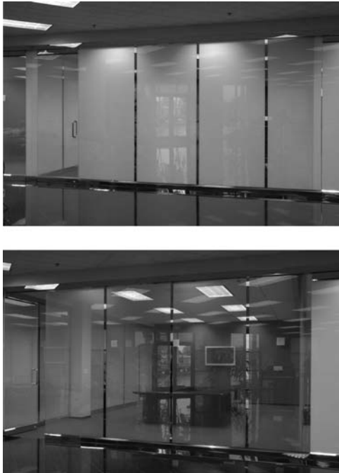
Fig 3 Polyvision glass demonstrating glass that switches from opaque to clear at the touch of a button. Top image: opaque (power off). Bottom image: clear (power on). Side rooms could be constructed using this glass. (Reproduced with permission from www.polytron.com.tw , December 2008.)
